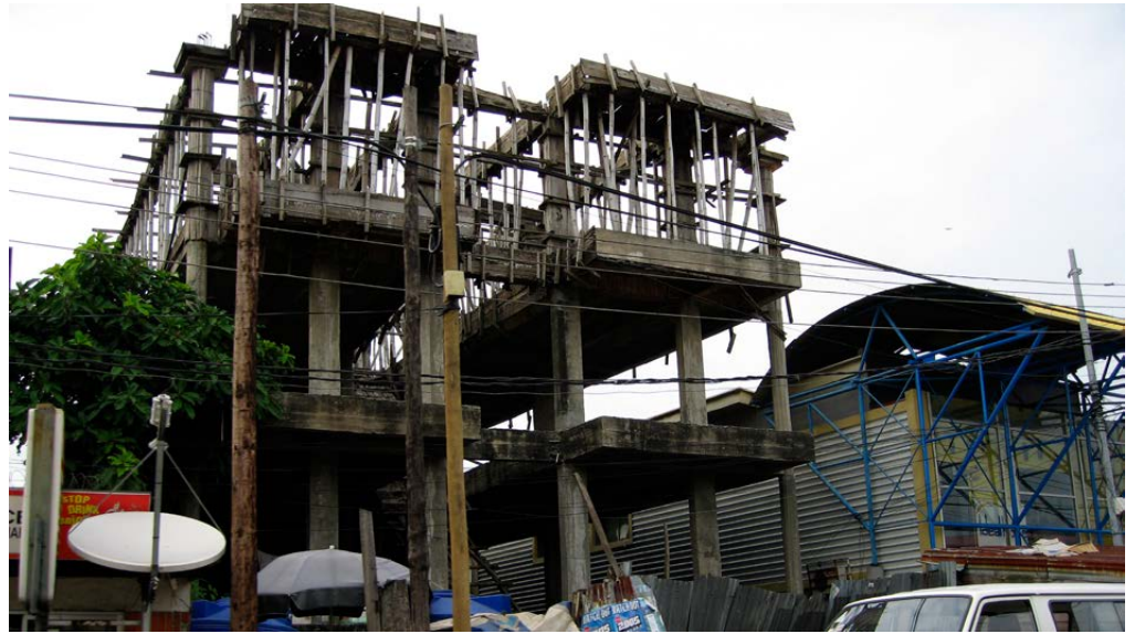
A building under construction in Lagos, Nigeria.
